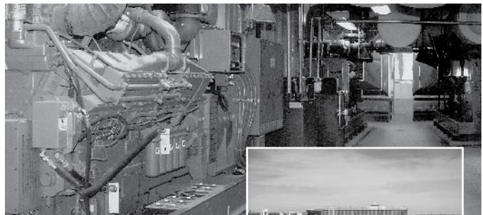
Four 1500 kW Cummins Power Generation generator sets provide backup power to the main terminal at Minneapolis-St. Paul International Airport.
