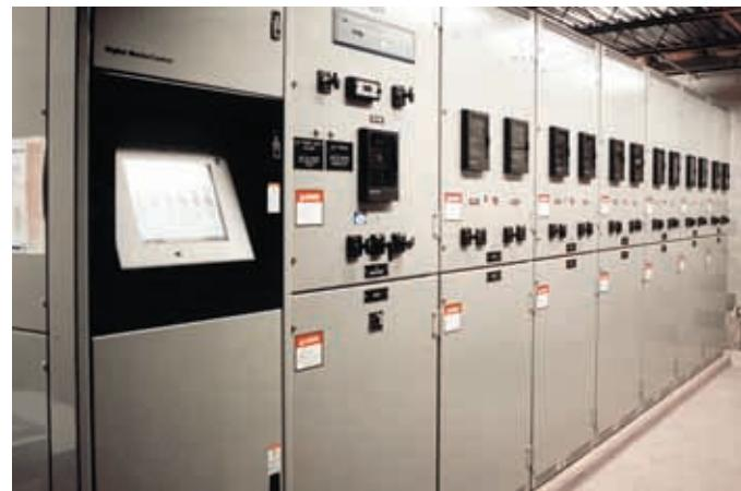
The system features digital master controls and parallel operating gear from Cummins Power Generation for reliable and precise performance. Digital systems also occupy 25 percent less floor space than traditional analog-control systems.
