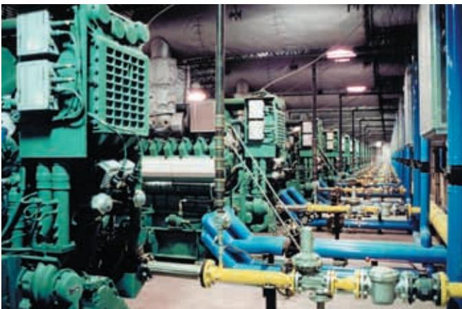
Twelve Cummins Power Generation lean-burn gas generators are operated in an interruptible mode during peak demands, essentially removing 21 MW of load from the TVA power system when running.
