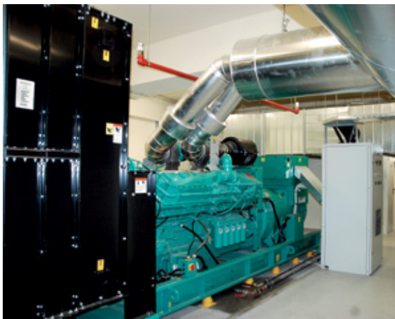
Ergotrak handled the whole installation including piping and ducts
