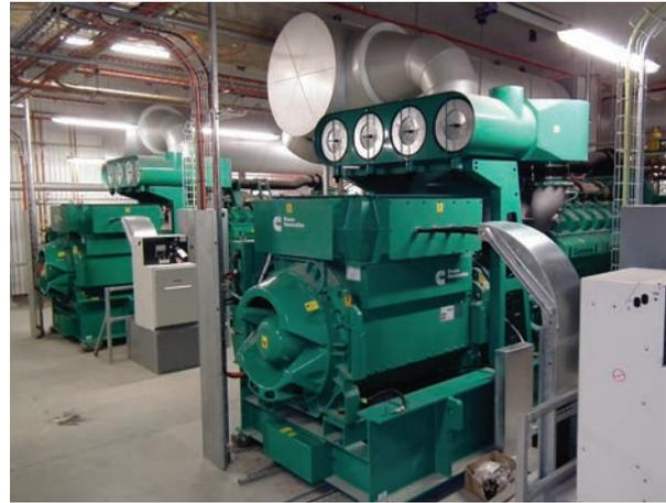
Two C2000 N5C generator sets with QSV91 engines installed at basement level
