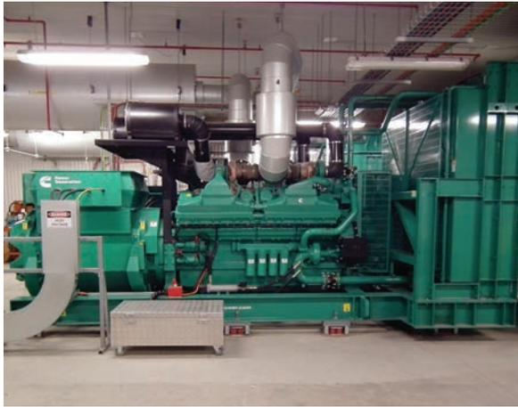
Emergency standby power is supplied by two 2500 kVA C2500 D5A generator sets with QSK60-G9 diesel engines
