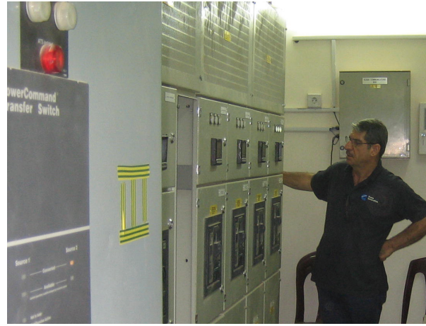
The power station operates automatically with the generator sets in parallel
