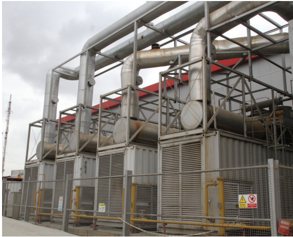
The NBC Ikeja site employs four 1750 kW Cummins generator sets
