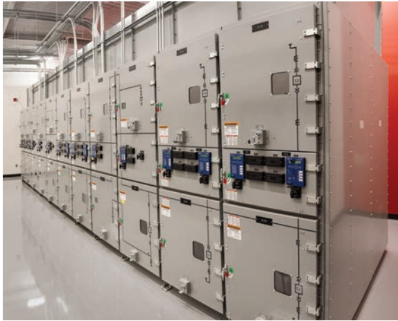
In addition to providing interruptible and standby power, the Cummins 5 MW power system is used for customer demonstrations
