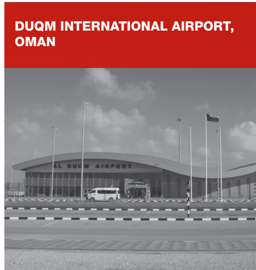
Duqm Airport relies on Cummins backup power to keep its operations flowing smoothly
