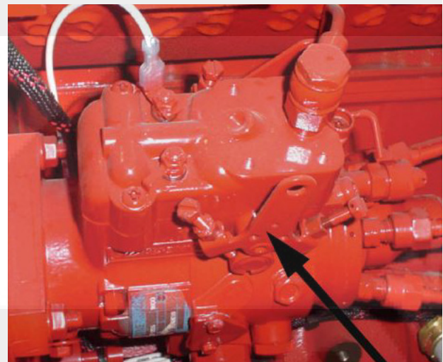
Figure 5-3 Fire Pump Drive Engine Throttle Bracket
