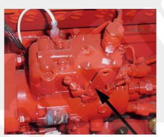
Figure 5-3 Fire pump drive engine throttle bracket
