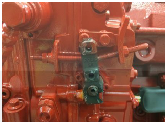
Figure 5-3 Fire Pump Drive Engine Threaded Linkage Rod
