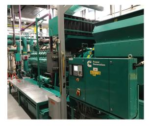
The engine exhaust passed through an external steam boiler to produce 100 psi of steam which was utilized by the university campus. The second path of thermal recovery was achieved in the form of hot water. The heated engine jacket water passed through a plate and frame heat exchanger supplementing hot water to fulfill all needs on campus.
