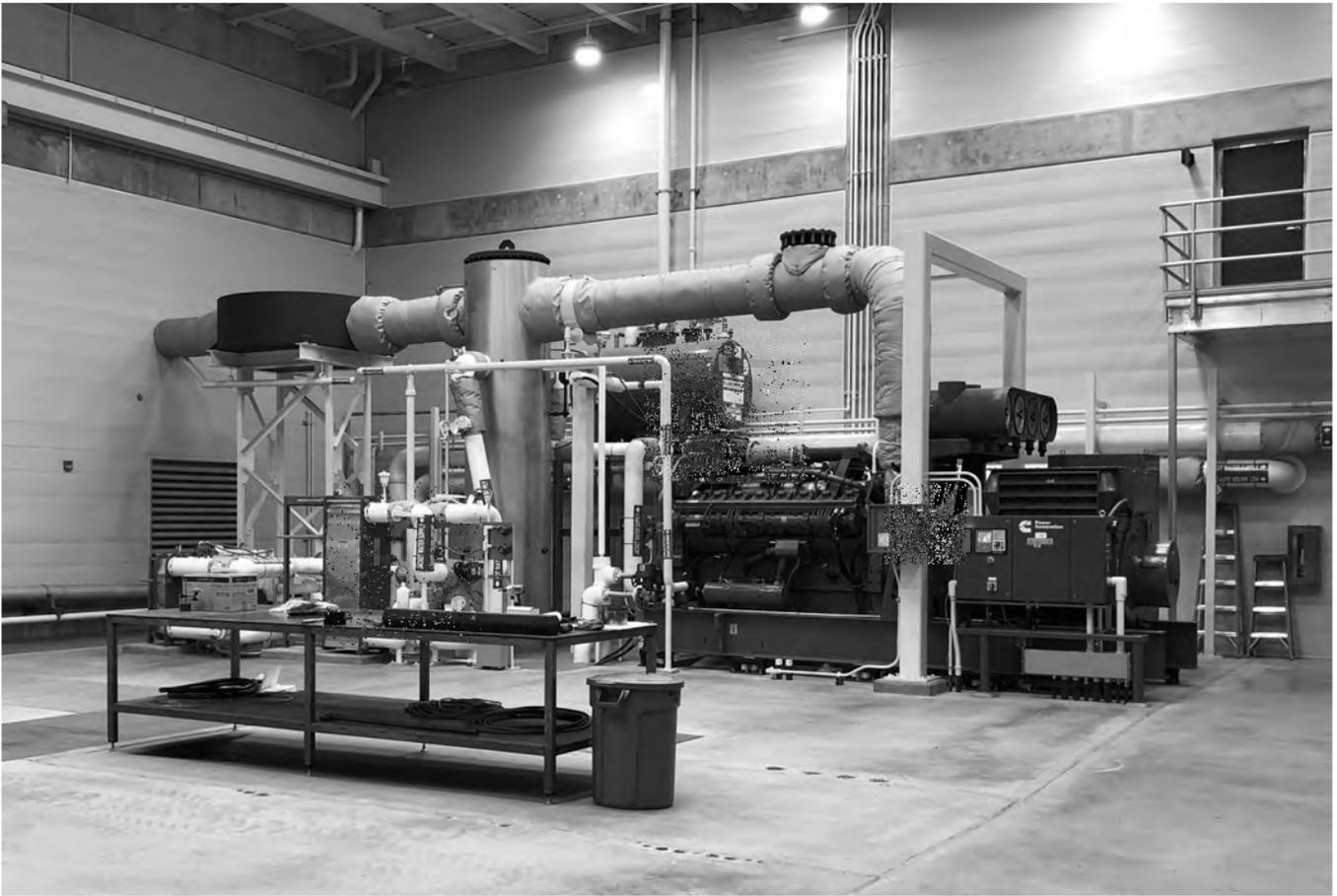
The QSK60G gas generator range offers a fully integrated power generation system which utilizes state-of-the-art technology to result in the optimum performance and efficient use of fuel needed for the facility's cogeneration needs. The treatment facility, as a by-product of its digestion process, produces approximately 300,000 cubic feet of methane gas per day. This excess gas is utilized to power the generators which, on average, supply 50-60% of the plant's electrical needs.
