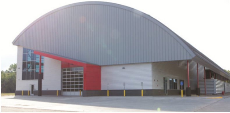
FIGURE 1 Outside view of Acoustical Technology Center (ATC), located at south side of the main plant of Cummins Power Generation at Fridley, MN, USA.
